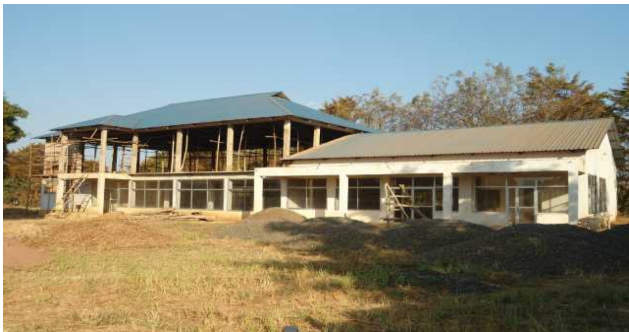
Picture 8. Modern library under construction at Kasulu town
