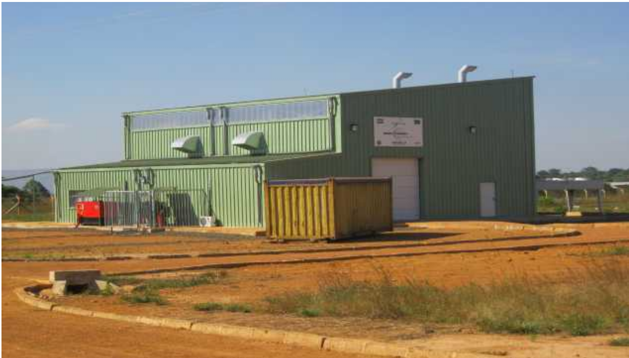
Picture 6: Electrical plant at Kasulu Town Council
